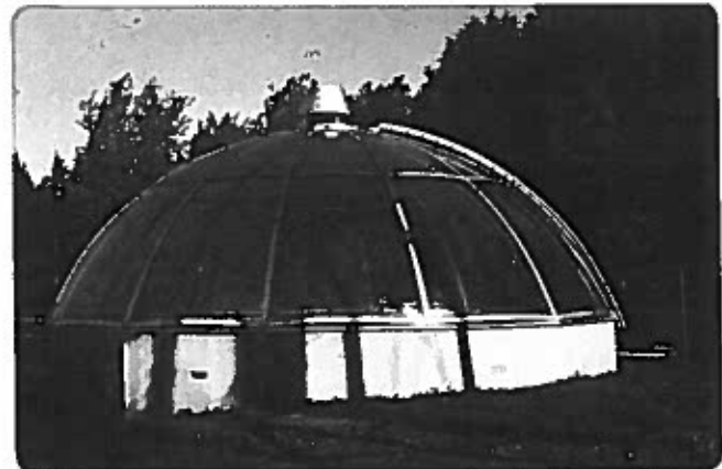
PRINCETON, MAINE; MODEL CH Plant covered with a plastic dome for Winter operation
