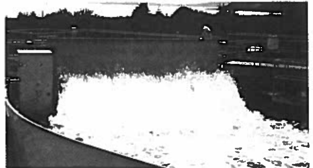
CENTRAL SAANICH, B. C.; MODEL MM A 17' Magna Rotor operating 10'-0" liquid depth
