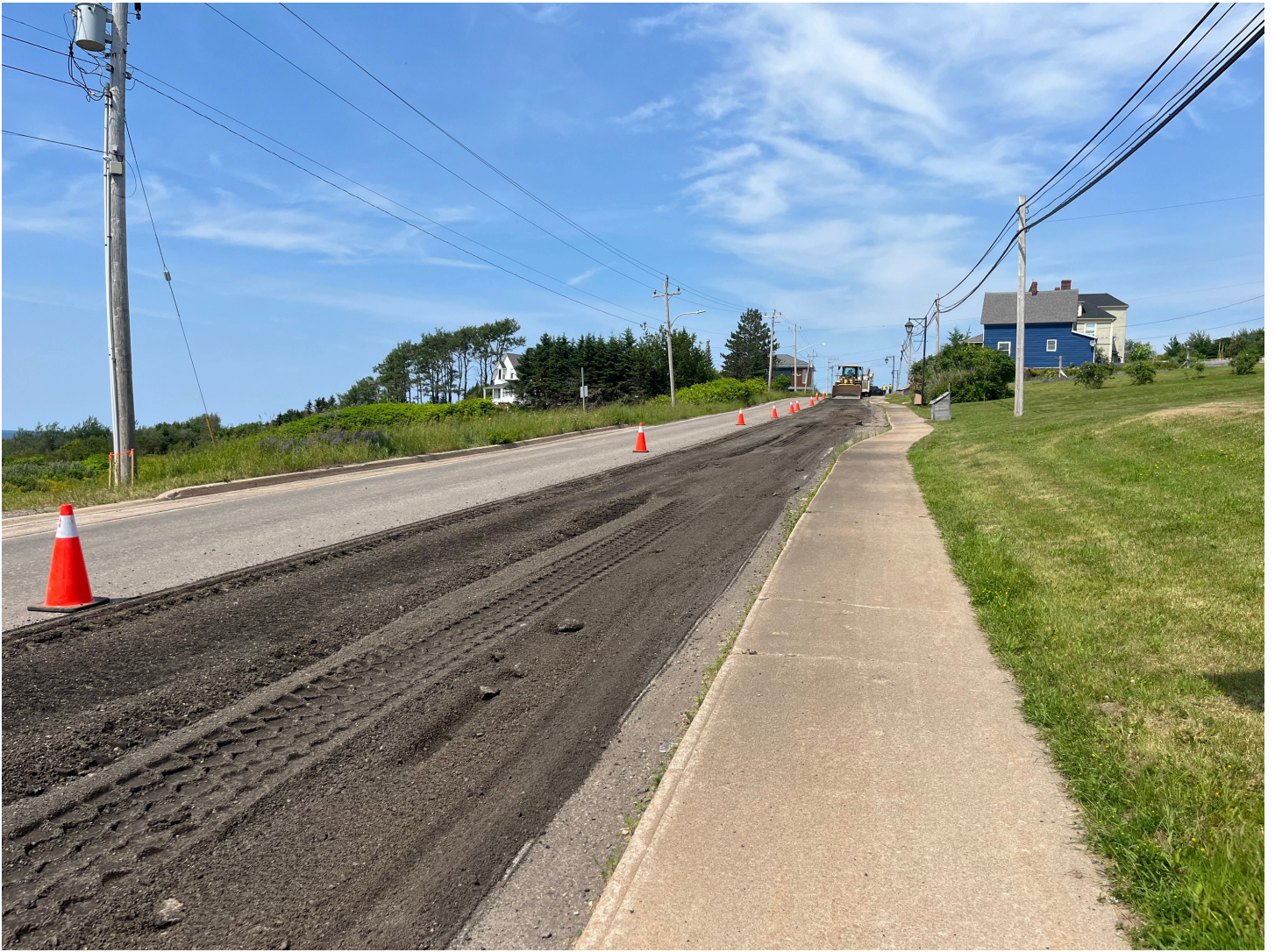
Pictured above: Asphalt on Central Avenue following pulverising on July 9, 2026.
