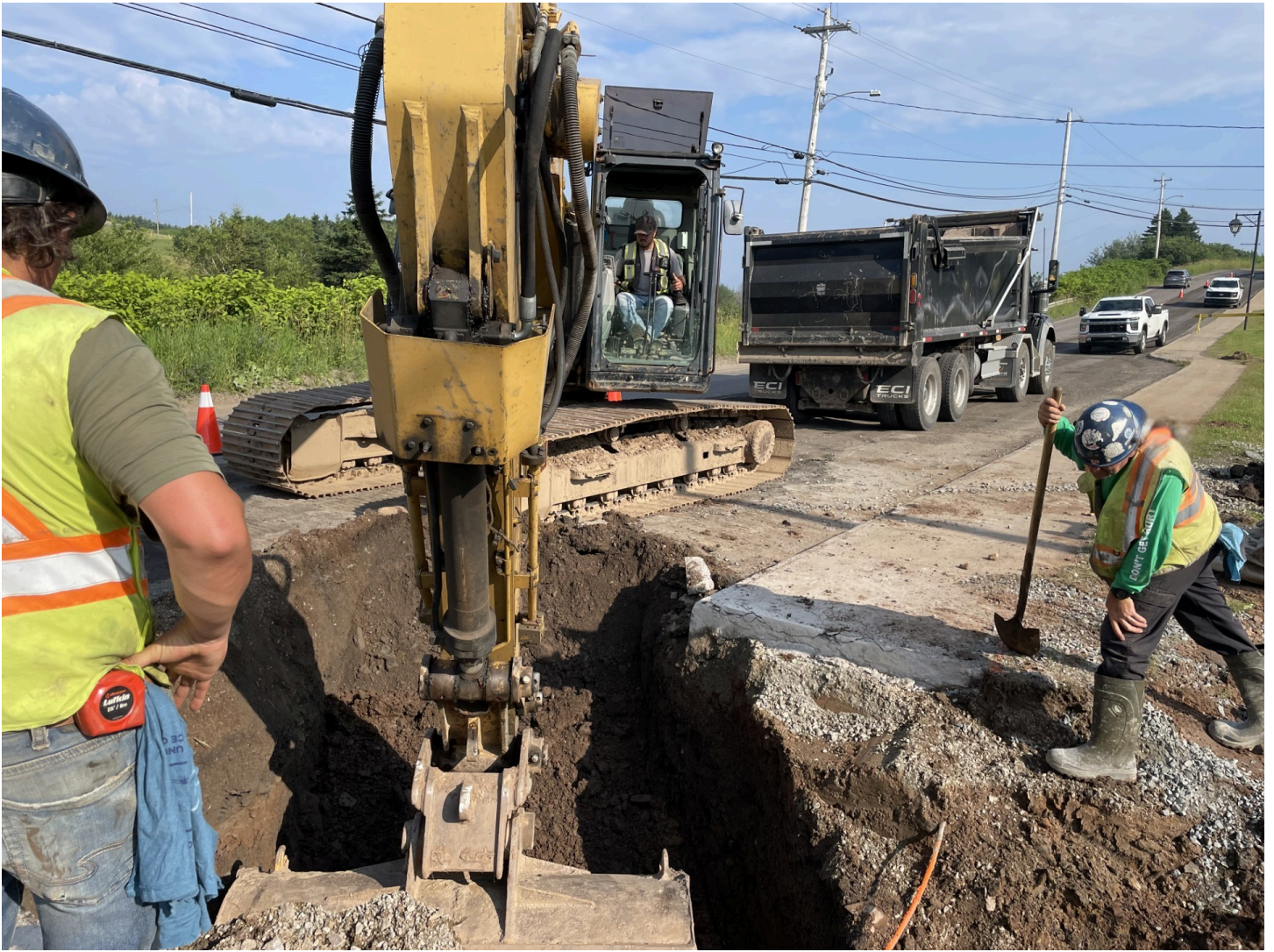
Pictured above: On July 15, workers continue to make progress towards replacement of the wastewater lift station.
