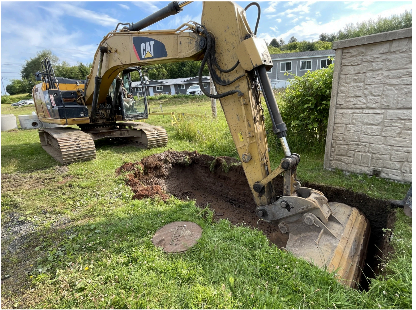
Pictured above: An excavator digging for the replacement of the wastewater lift station near the Shean Trail Crossing on July 13.
